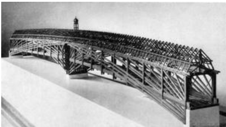
Figure 2: Model of the main structural members of the Rheinbrücke in Schaffhausen, CH.
