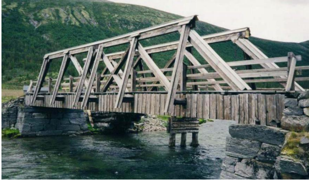
Figure 13: Ponte Timber bridge over the river Finn at Loom, Norway. Note the meticulous protection of the building structural load-bearing parts. The bridge is more than 100 years old.
