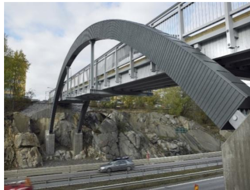
Figure 14: Left: principle of “mechanical” protection of a timber load bearing member by means of wearing planks at sides and metal sheet on top. Right: example of a timber bridge near Stockholm, Sweden; note the mechanical protection of the arches and of the deck.
